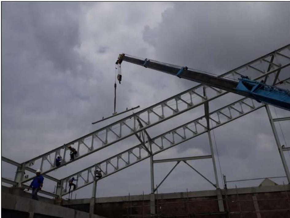
**Gambar Proses Erection Steel Structure**
