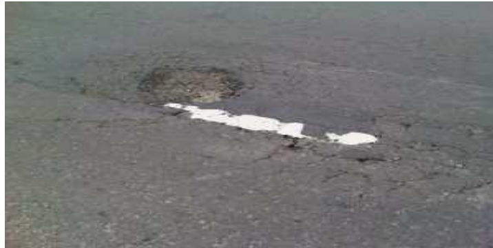
Gambar 2.13 Lubang ( potholes )
