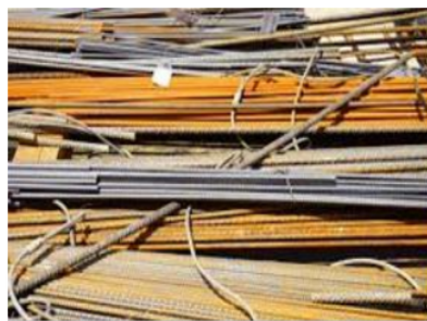
Figure 1. Corrosion in reinforced steel.
