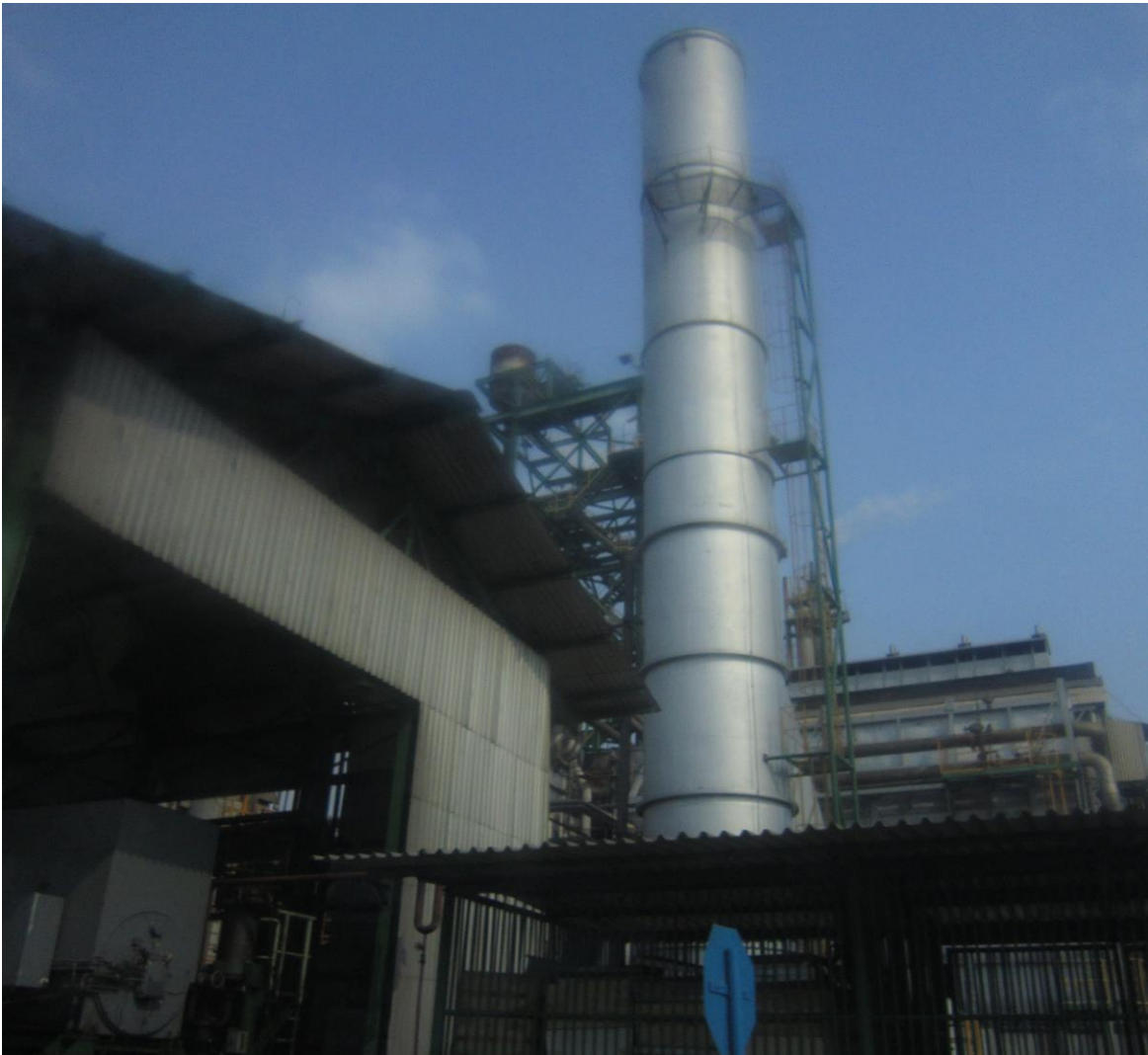
Gambar..... Pusri Effluent Treatment (PET)
